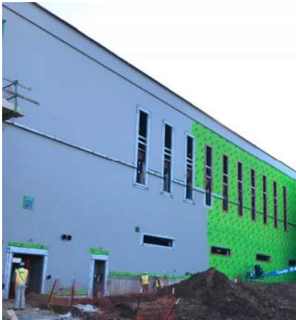
Liquid applied membranes w/ sealed joints
