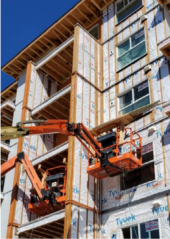
Wood strapping over mechanically attached housewrap WRB
