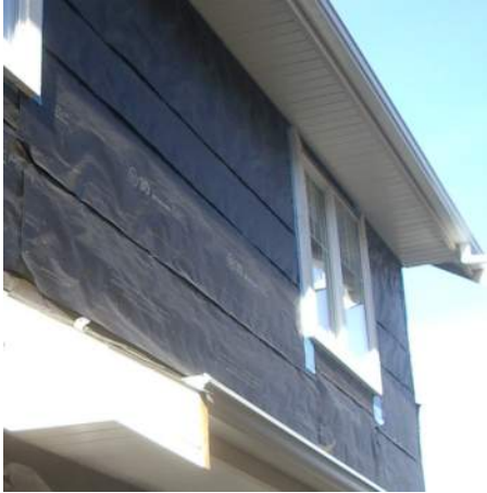
Building paper w/ lapped joints
