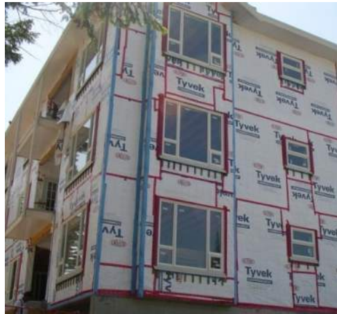
Mechanically attached house-wraps w/ taped joints
