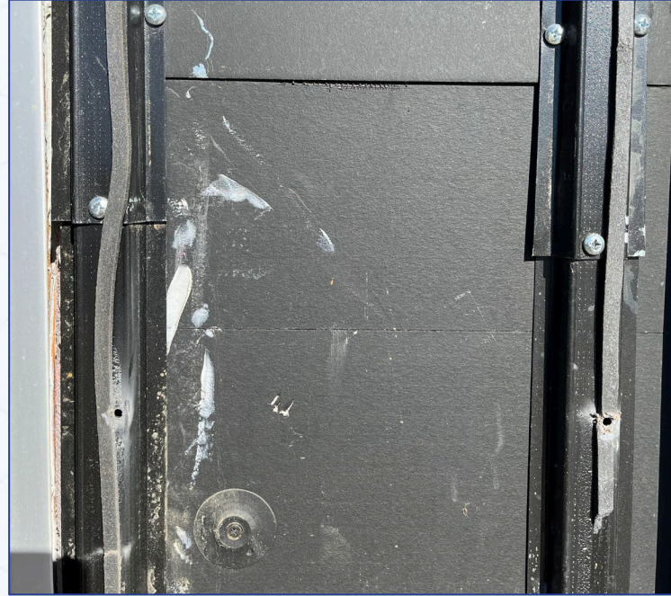
Overlapping profiles and protruding screw heads
