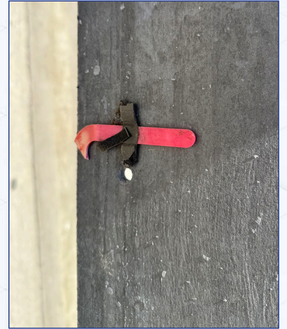
Plumb the profiles, not the panel
